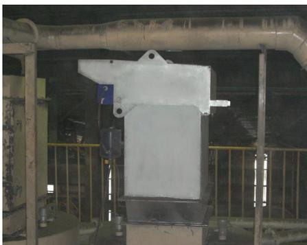
Silo venting system for additive silo, *Foundry Industry*
